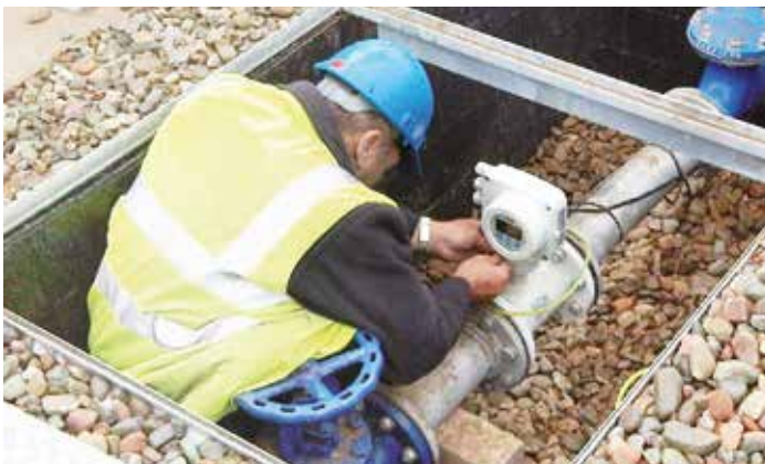
WaterMaster unit being installed on water line
