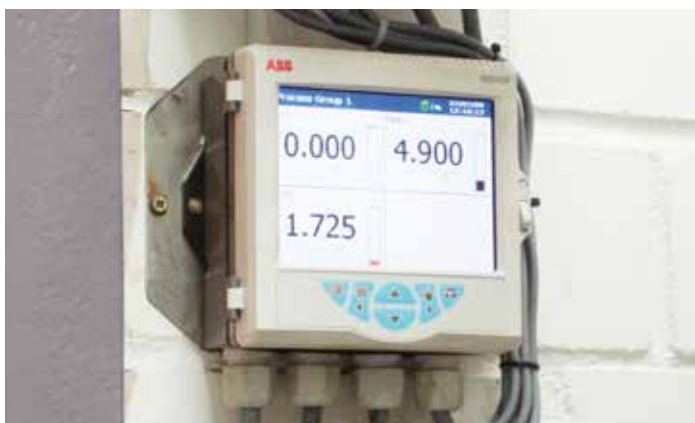
Remote mount videographic recorder SM500F monitoring effluent flow
